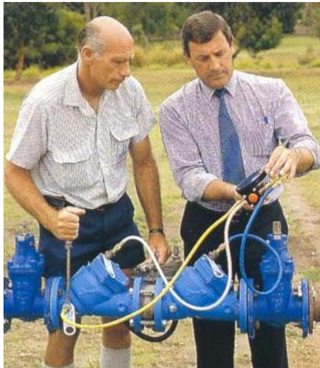
Figure 16.4: Commissioning a backflow prevention device
