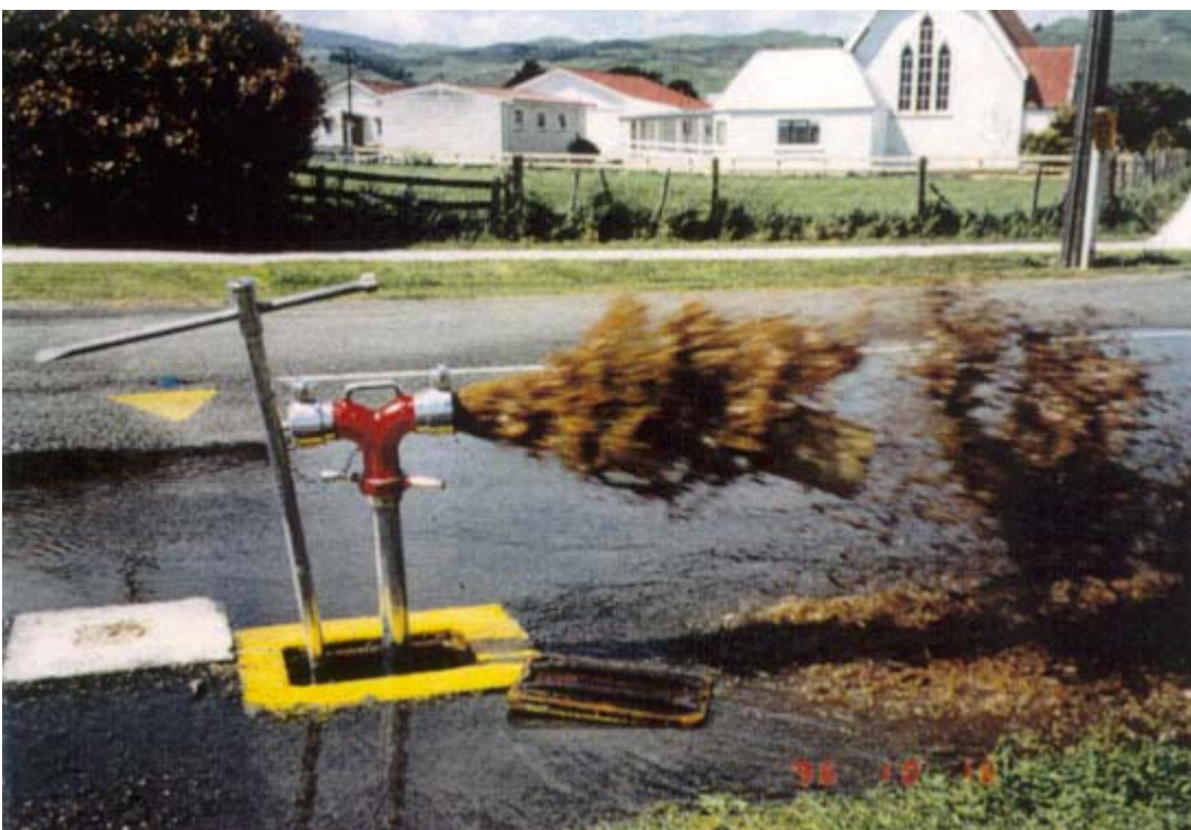
Figure 16.3: Fire hydrant standpipe being used to flush a water main
