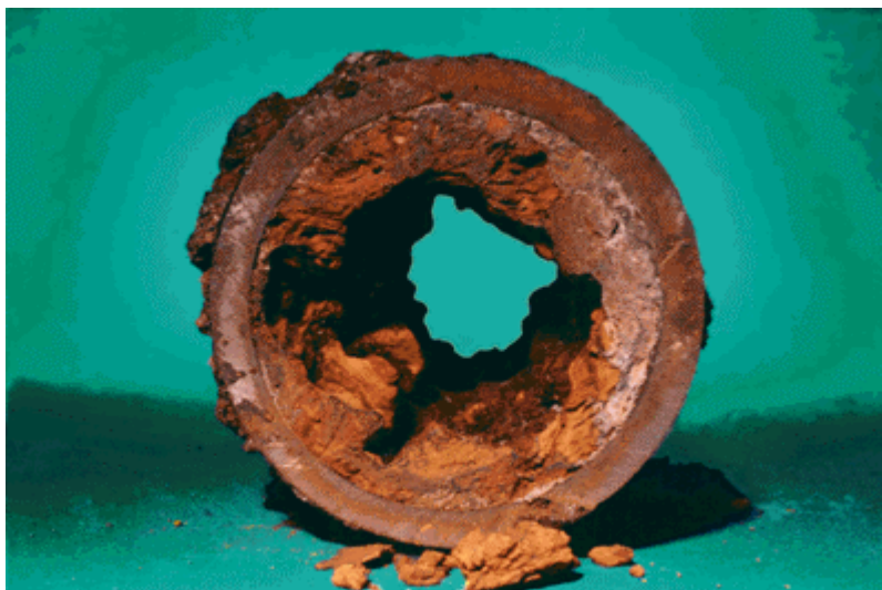
Figure 16.5: Example of corroded water pipe
