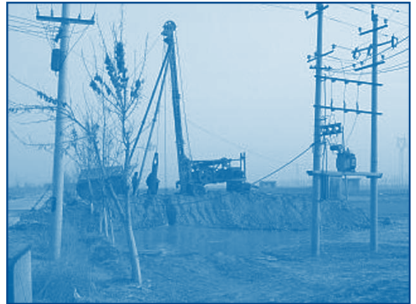
Zhongwei County – new well development
