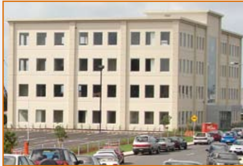
The Waimarino building
